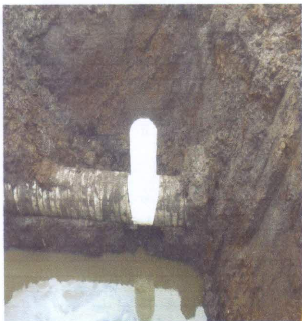
FIG.3 SHOWING SPILL POINT (AFTER REPAIR)
